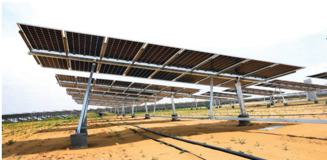
Figure 11 Sketch Map of Installation of Bifacial Module
